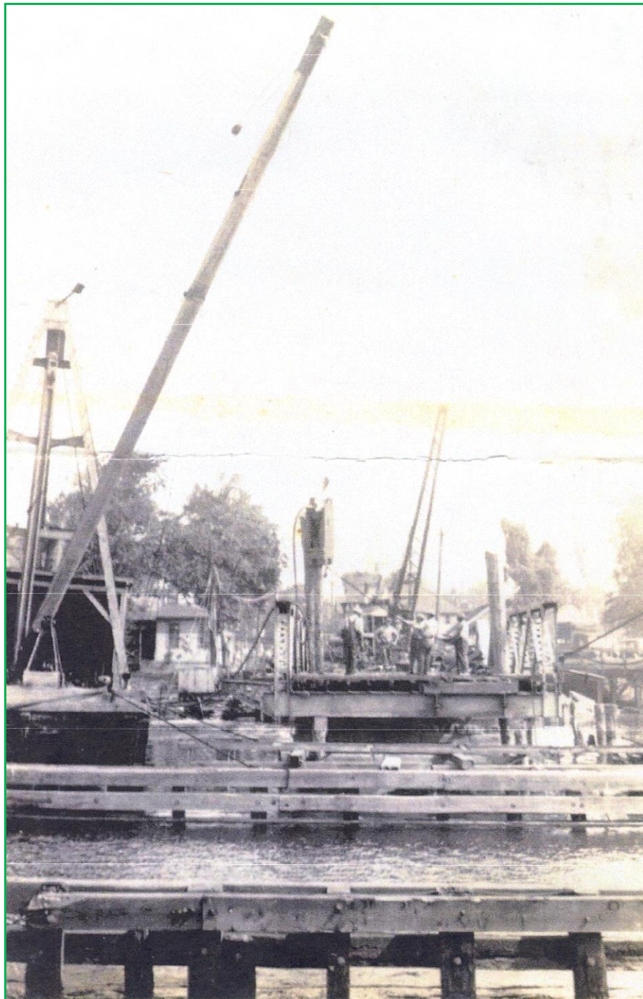
steel sheeting being driven for the new bridge
