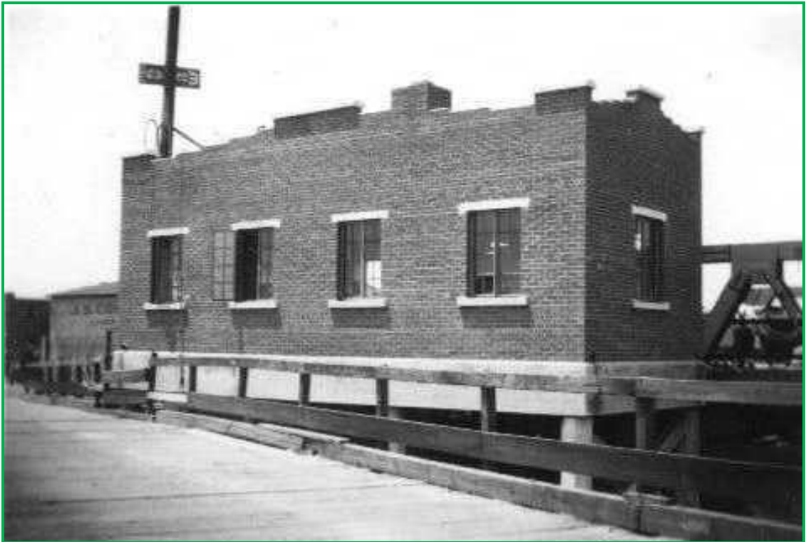
the eastern (back) side of the Bridge Tender's building c1935
