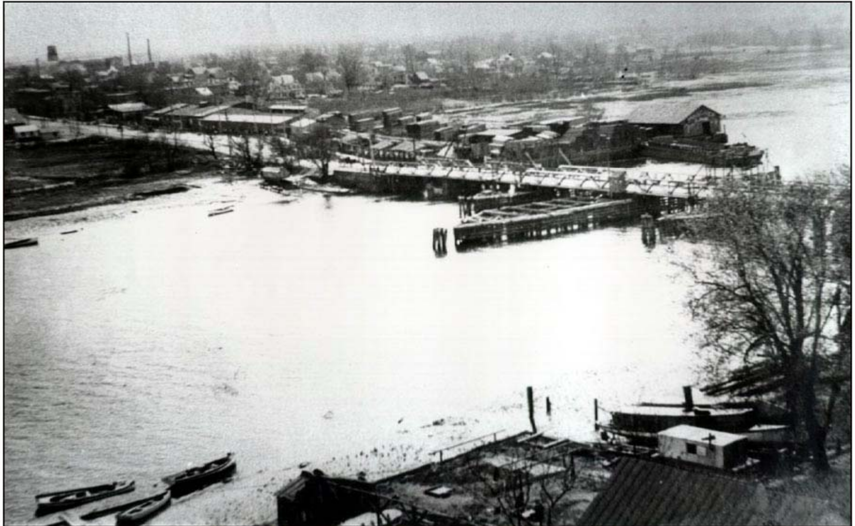
View Looking Towards Riverside
