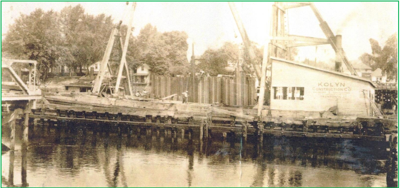
steel sheeting being driven for the new bridge
