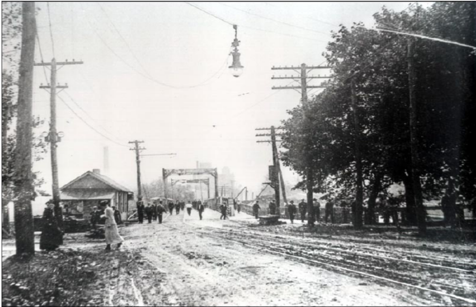
View Looking Towards Riverside Note Workers Returning From Watchcase
