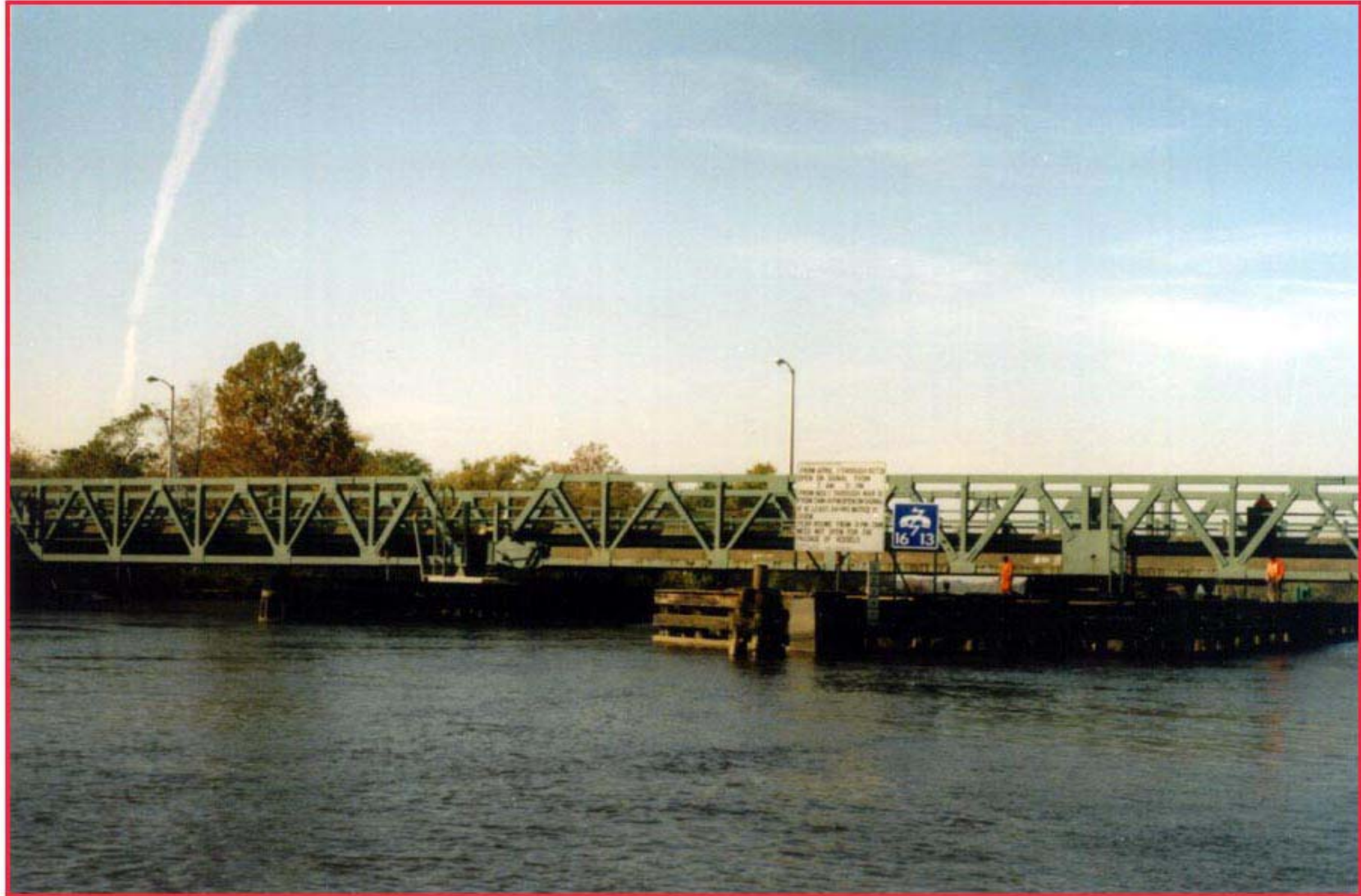
Swing Span Shown In Closed Position Photograph Taken in 1993
