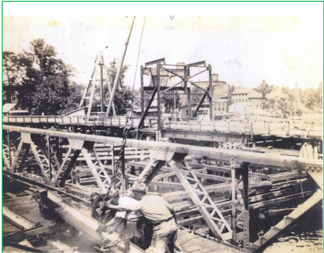
demolition of the existing 1901 second bridge at the same site
