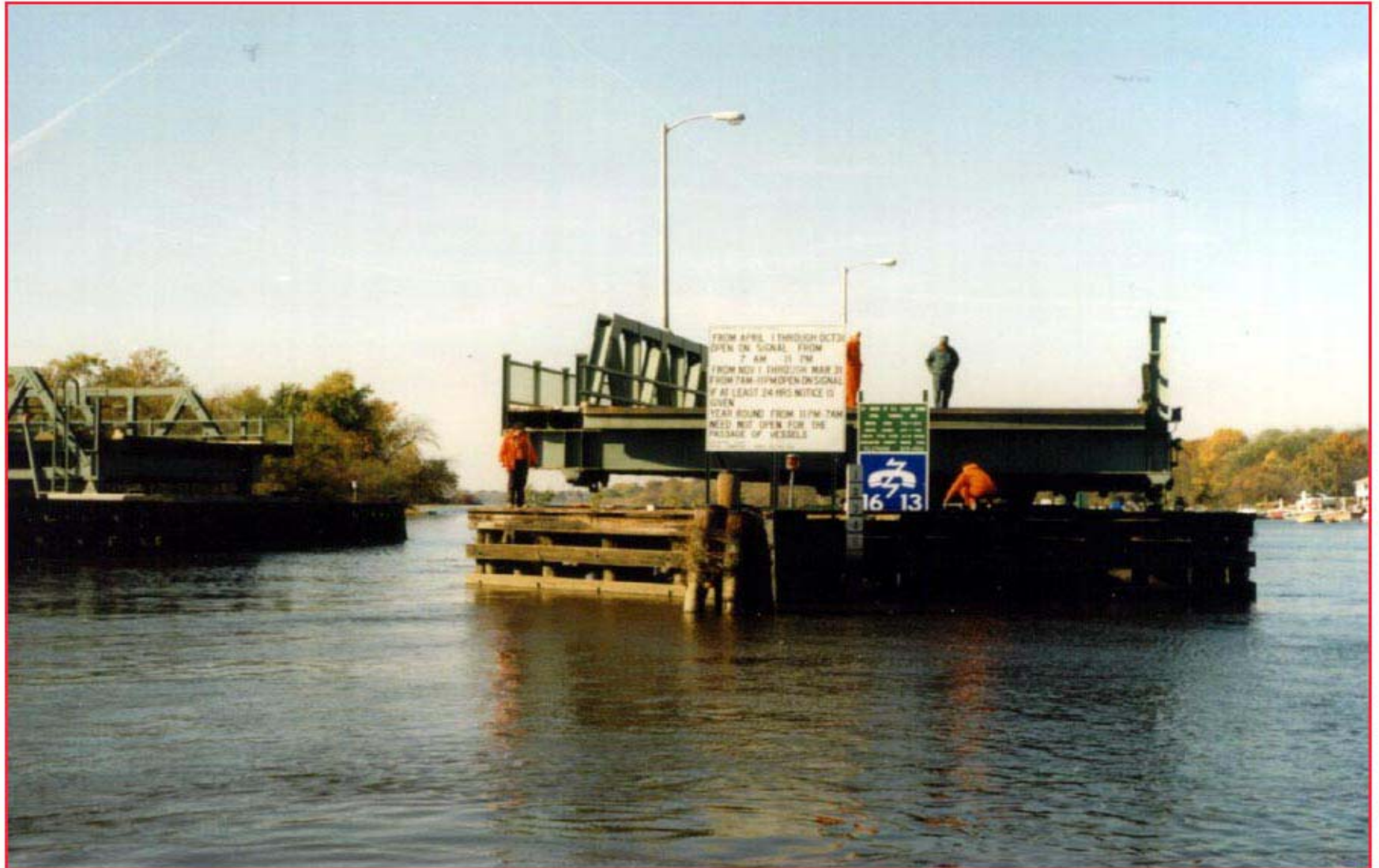
Swing Span Shown In Open Position Photograph Taken in 1993
