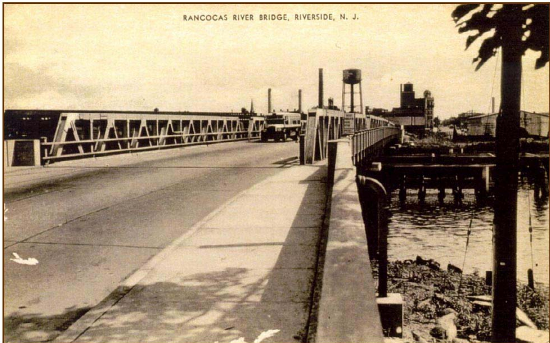
Postcard of Riverside-Delanco Bridge Date Unknown (sometime after 1935 when bridge was built)
