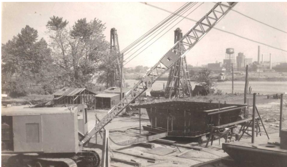
A steel ship, probably the 65-foot, 60-ton US Army Ferry Maj. Carroll Edgar, under construction at Robins Shipbuilding in Delanco. It was launched September 9, 1941 and put into service at Ft. Slocum, NY.
