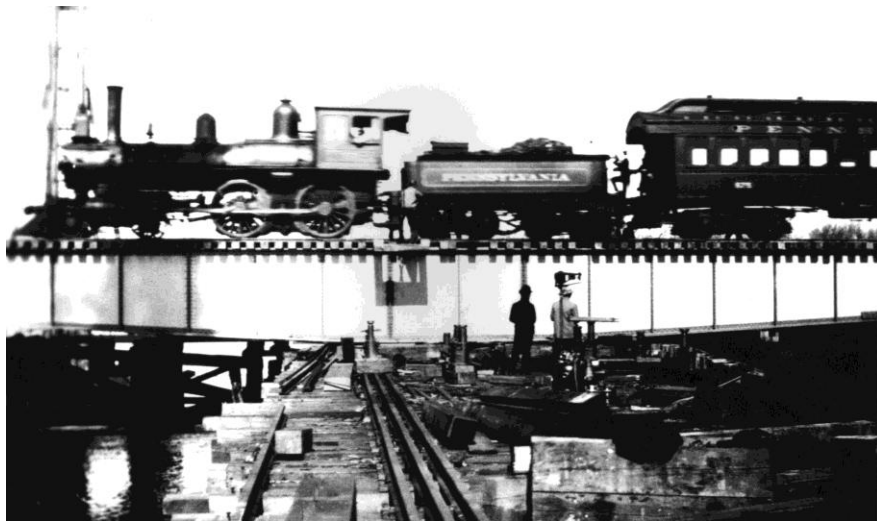
This photo is reported to be of the first train to cross the newly completed turntable bridge on the Rancocas Creek in 1906. The span was moved to Delanco from its former location on the D&R Canal.
