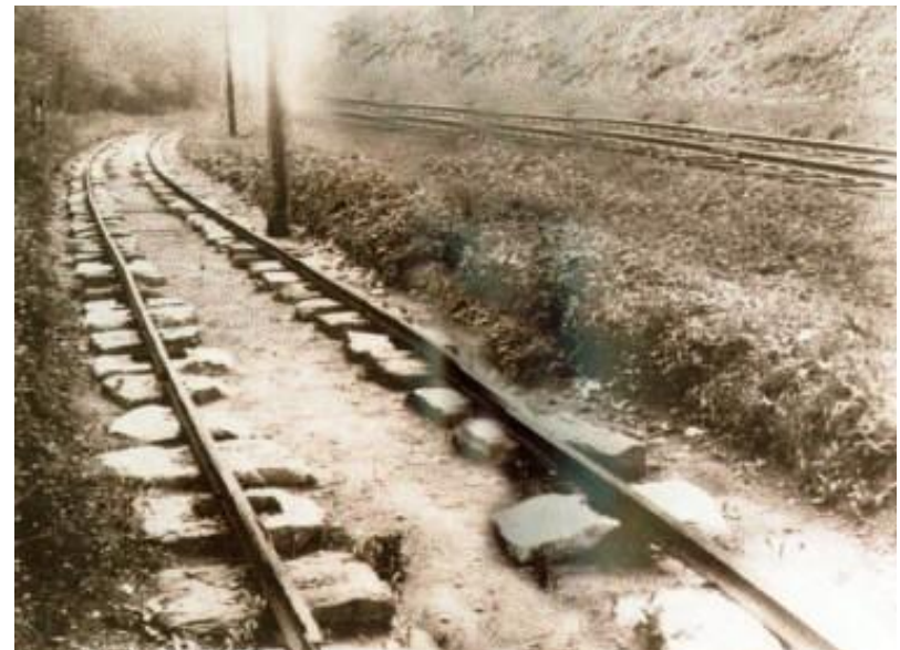
Photo of original stone sleepers and rails adjacent to a modern rail and wooden tie roadbed set in stone ballast.
