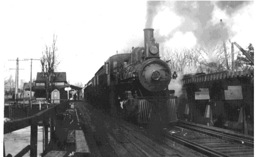
A Pennsylvania Railroad engine heading south over the Rancocas Crossing bridge. Note the newer, higher bridge under construction to the right and Delanco Station to the left.
