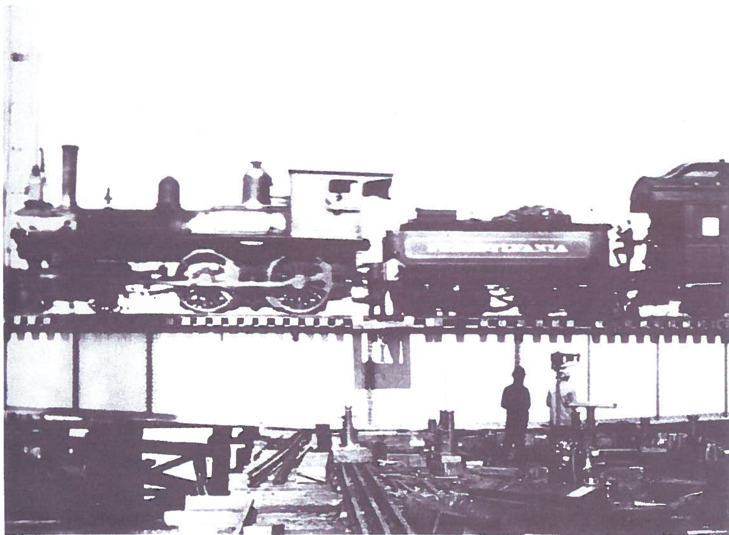
THE FIRST TRAIN crosses the new swing bridge over the Rancocas Creek between Delanco and Riverside in 1906. In the foreground, loose timbers lie on the barge, which was used to transport the center span,
