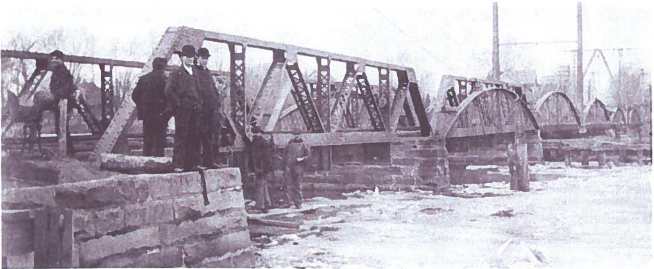
NEW PEDESTRIAN and automobile bridge over the Rancocas is shown being constructed in 1901 inside the old one. The new bridge shown at left is a Warren Truss Bridge replacing the old rounded Bow Truss
