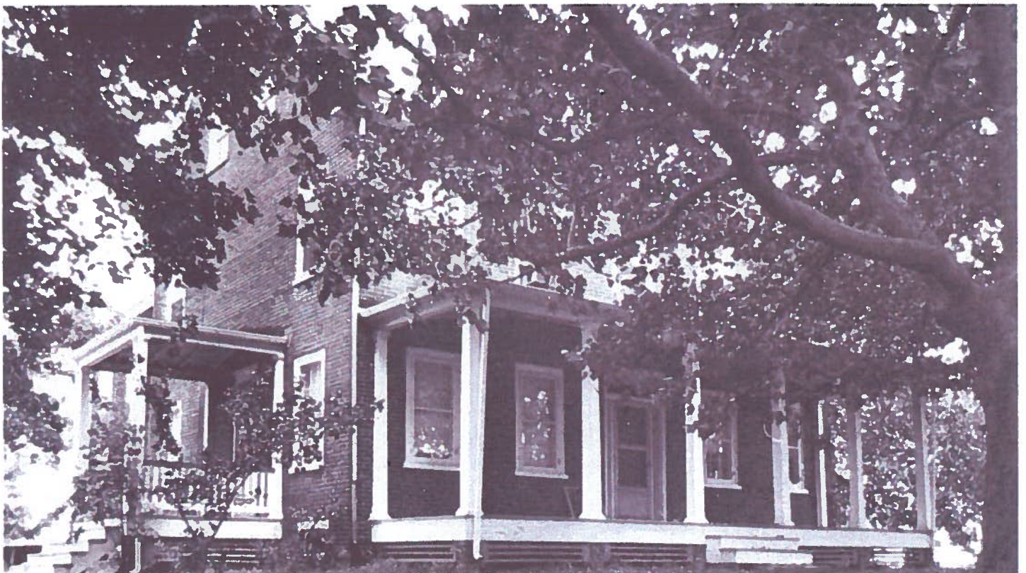
THIS IS the Stanley Russ home, located on the Rancocas Creek. The original structure would have been
