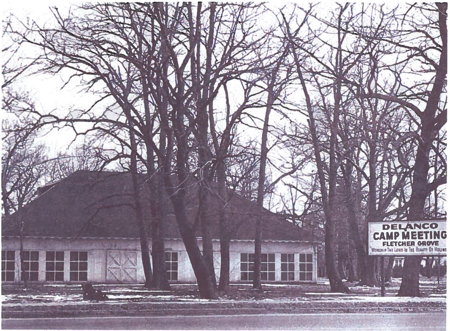
THIS IS ONE of the last photographs taken of the Camp Meeting auditorium before it was demolished in 1974 to make way for a shopping center. The view is
