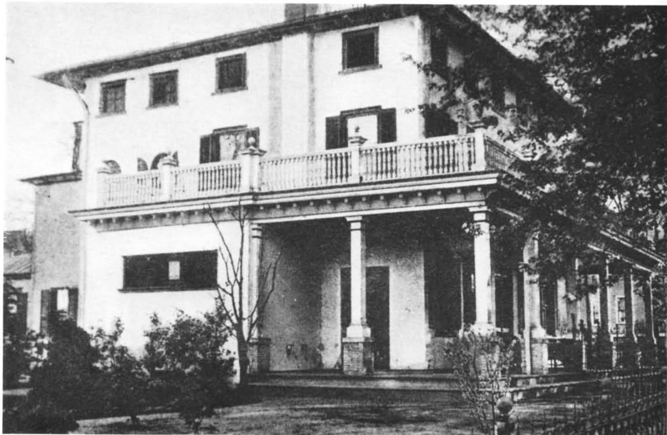
ZURBRUGG'S first residence, at the corner of Taylor and Franklin Streets in Riverside, became the first hospital. Later, it was used as quarters for the nursing staff
