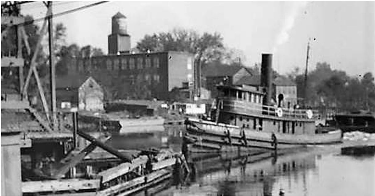
This photo, taken some time after 1912, shows the orientation of the original frame factory building and its addition in relation to the newer frame factory. Borel's boatshed is to the left of the factory. In the foreground is the steam tug Rancocas with a barge in tow, heading downstream toward the swing bridge. This was a busy time for commerce along the Rancocas Creek, when the waterway was a major asset to the growth and prosperity of Delanco. Photo from the Delanco archive.
